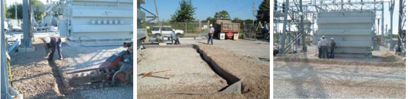
Above ground dike install for large facilities and equipment
