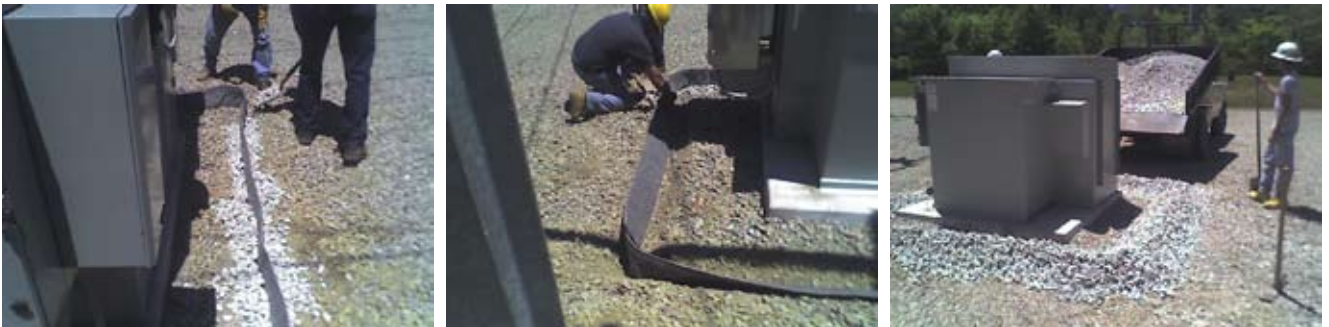
Pad mount install for smaller containment
