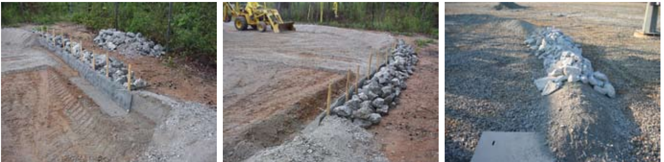
Water gate install to process water
